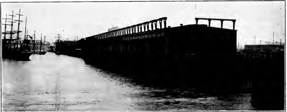
Harbor view of Portland's municipal Dock No. 1. Length, 955 feet; width of dock shed, 100 feet; width of dock, including platform, 122 feet. Slip in foreground is 120 feet wide and 484 feet long, with 60-foot uncovered dock adjoining on the south.
